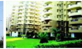
Vigyan Vihar, Gurgaon completed
