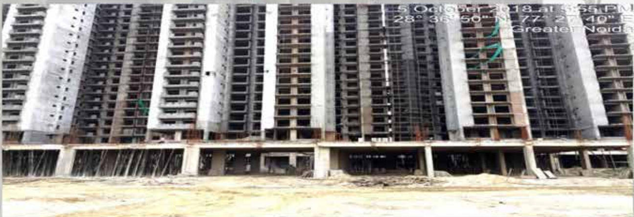
T-7 TO T-9 REAR SIDE NON TOWER CENTRAL AREA SLAB CASTING ON PROGRESS
